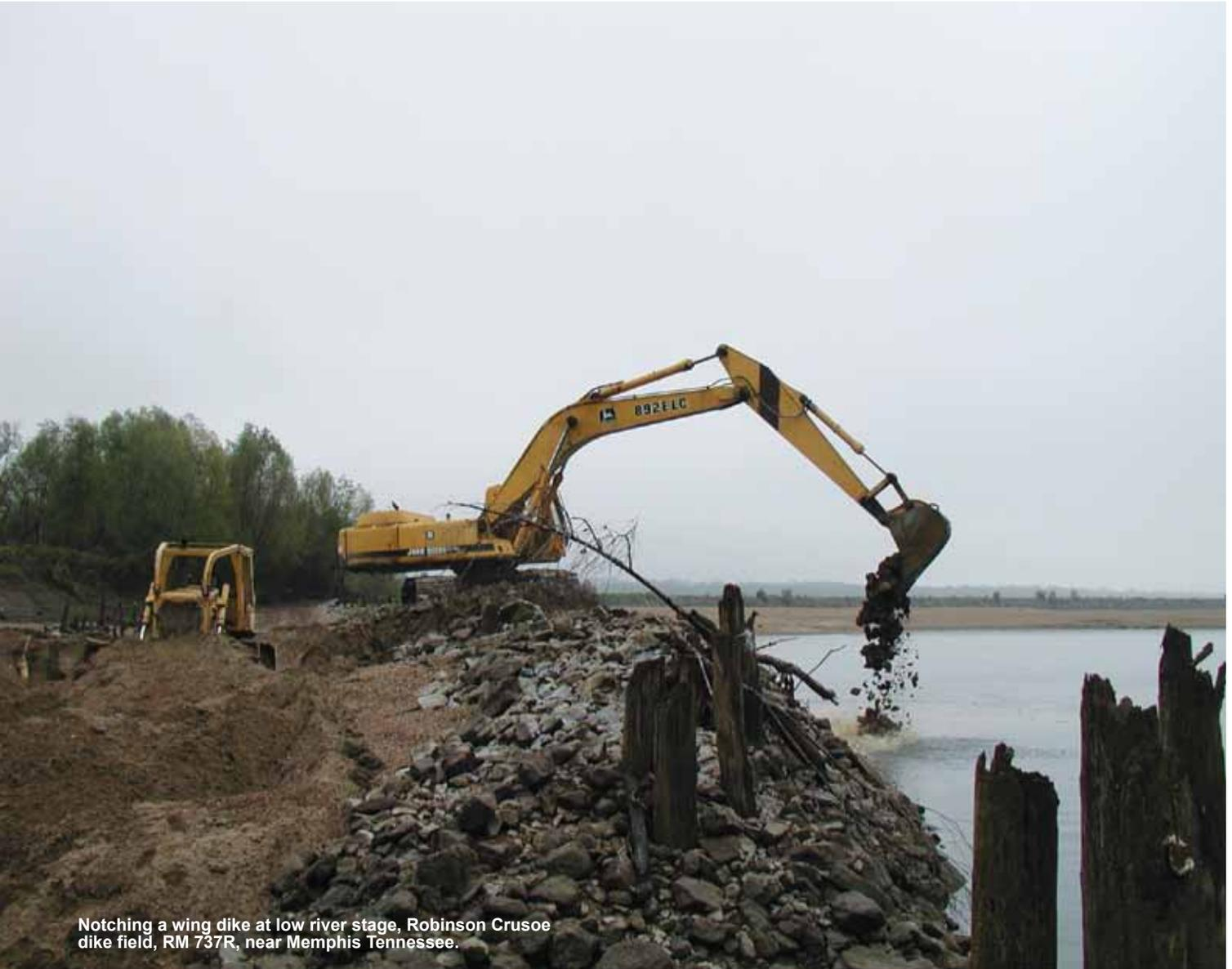
Notching a wing dike at low river stage, Robinson Crusoe dike field, RM 737R, near Memphis Tennessee.
